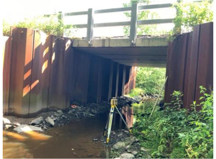
An example of abutments on Wynkoop Road. Local ID: LEW_021
