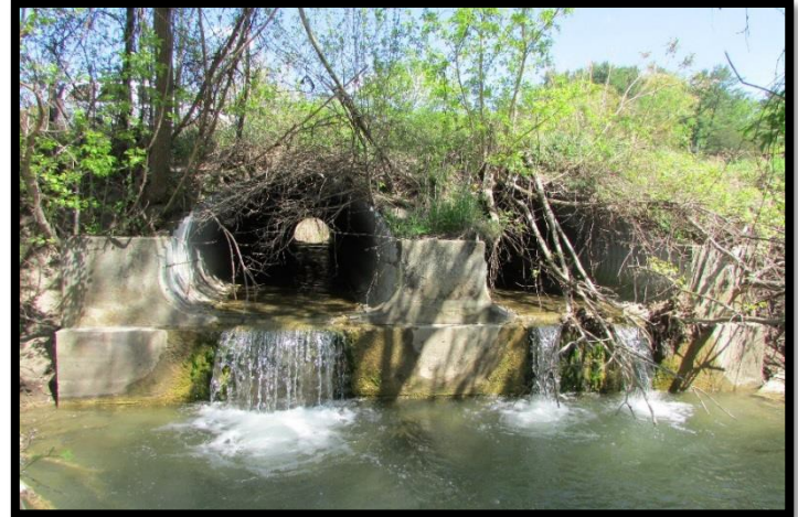
Culverts such as this these can constrict the natural flow of the stream, have a perched outlet that only strong swimmers can jump and contain no natural streambed. Many culverts and dams fragment
