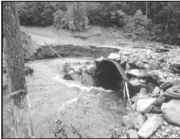
Bridge and Culvert Assessment
