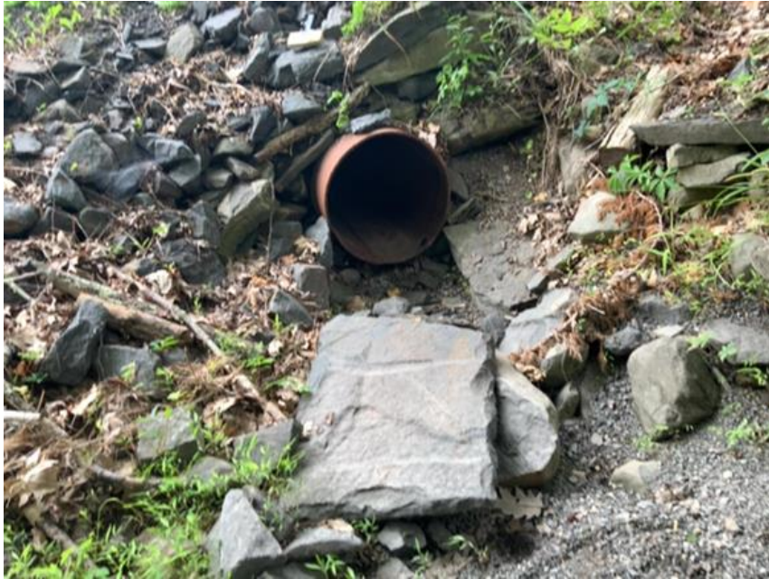
An example of a culvert with an outlet drop on Atwood Road. Local ID: LEW_031
